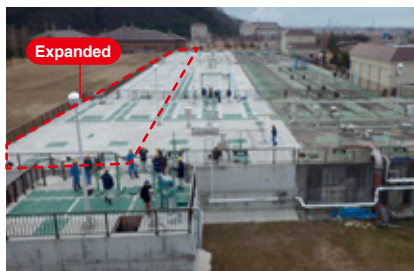
Photo: Expanded water treatment facility (Ishinomaki Water Treatment Center)
