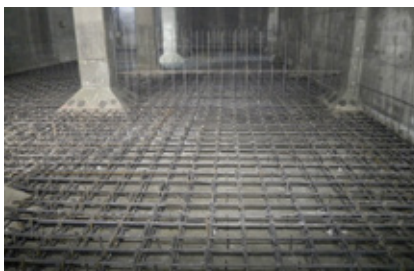
Photo: Fumotoyama No.1 regulating reservoir under seismic retrofit work
