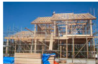
Photo: Support for new home building using the Miyagi quality wood
