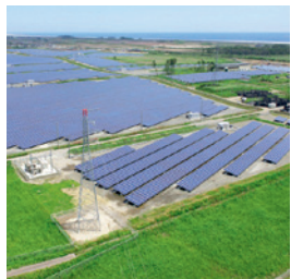
Photo: Mega solar power plant (Iwanuma City)
