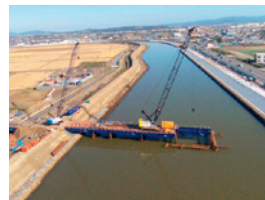
Photo: Construction of a temporary bridge linking piers on the Jokawa River (Higashimatsushima City)
